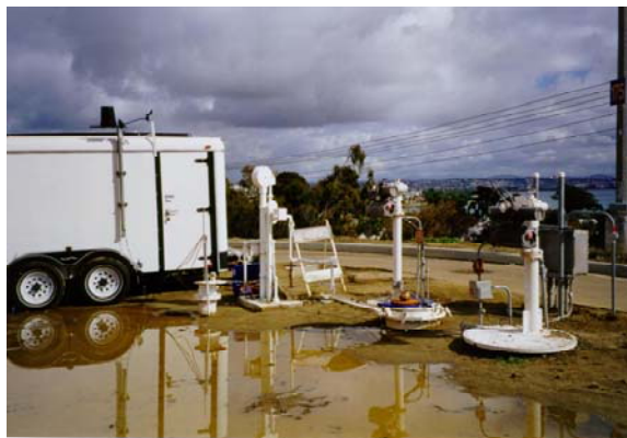
Figure 3. Tank 175 at the Point Loma Fuel Farm.
