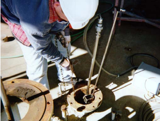
Figure 6. Top of the LRDP being installed in an 8-in. opening in a 50,000-gal UST at the Hunter Army Airfield.
