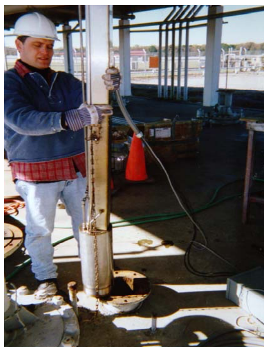
Figure 5. Installation of the LRDP in the 50,000-gal UST at the Hunter Army Airfield.
